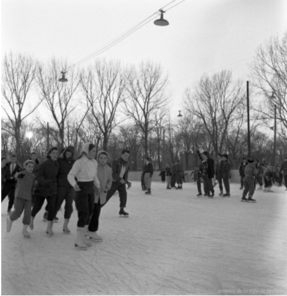
Skating facility, Parc Lafontaine.
