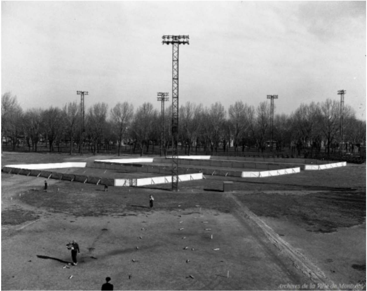
Construction of skating facility, Parc Lafontaine.
